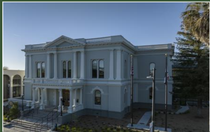
Willows Courthouse Post-Renovation
